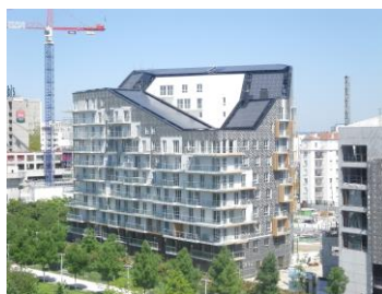
Figure 2 – Low-energy building in Paris' 17 th arrondissement (96 kW BIPV designed and installed by Sunvie).
